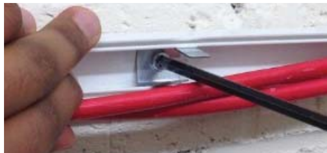
2. Slide clip under screw head and tighten
