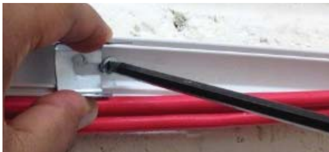
1. Pullout cables, slacken off screw
