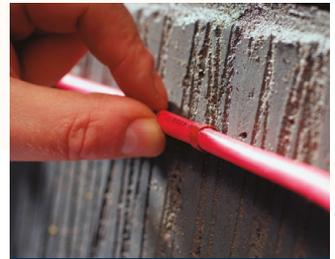
**3** Compress the LINIAN Clips legs and simply insert into the hole by hand.
