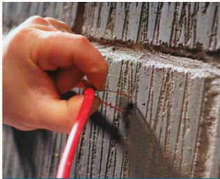
**2** Slide the LINIAN Clip over the cable, so that it is seated in the rounded area.
