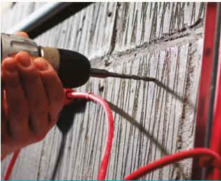
**1** Drill 5.5 mm diameter hole into the required material.
