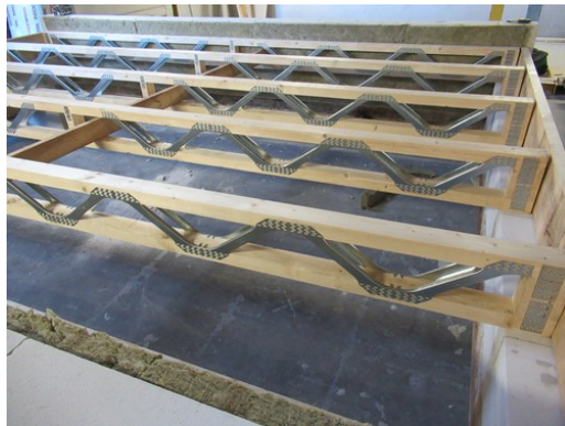
Photograph 2: Easi-joist® system during build up.
