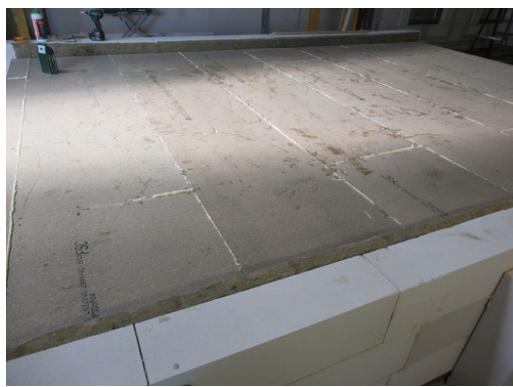
Photograph 4: Finished installation of the chipboards.
