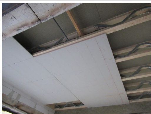
Photograph 6: Installation of the gypsum boards.
