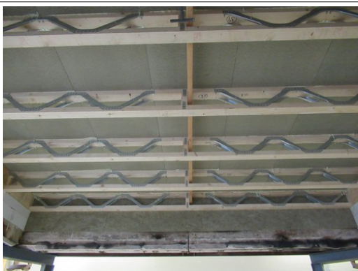
Photograph 5: Finished installation of the chipboards – view from underneath.
