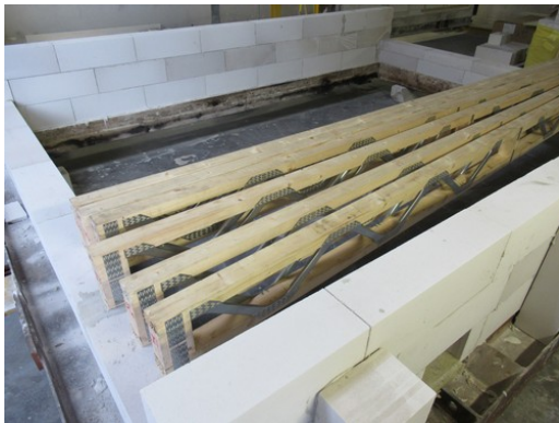
Photograph 1: Easi-joist® system during build up.
