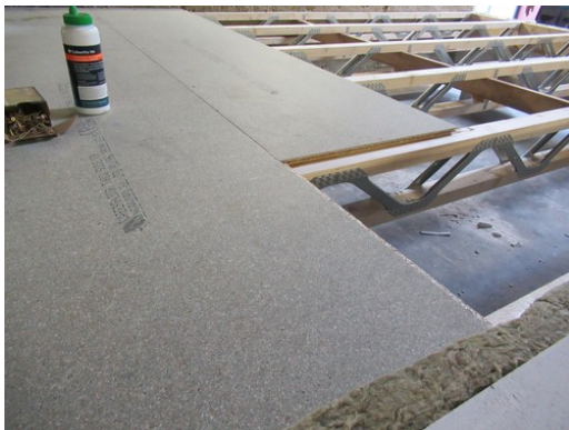
Photograph 3: Installation of the chipboards.
