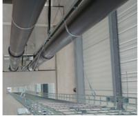
All hangers are supplied as ready-to-use kits with a length of wire rope and end fixing of your choice.
