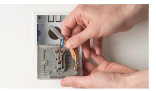
Place the brown wire (live) into the COM terminal, the switched live wire (blue/brown stripe) into the L1 terminal and the green/yellow wire (earth) into the separate earth terminal on the face plate.
