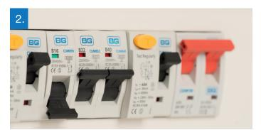
At the consumer unit, find the trip switch which protects the circuit and turn it all the way off. The indicator window should stay green.
