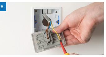
Make sure that the wires are fully inserted into the terminal and that no bare copper wire is visible. Tighten the screws securely onto the copper wire, not the outer sheeting.
