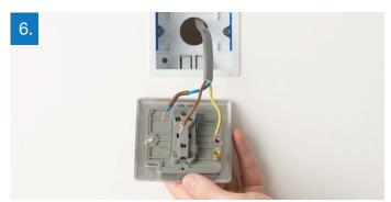
Line up the new switch and take note of where each terminal is located.
