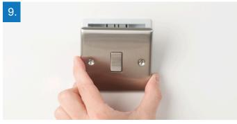
Gently press the socket back into place over the mounting box. Take care not to trap any wires between the wall and the socket.
