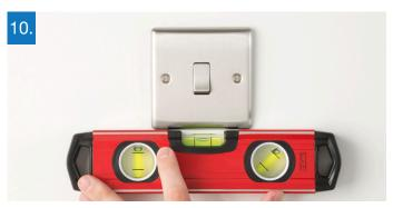
Insert and tighten the retaining screws provided. Use a spirit level to make sure that the socket is level. Restore the power at the consumer unit and test. For your safety, this product must be installed in accordance with local Building Regulations.
