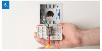
Unscrew each terminal to release the wires. You should now be able to remove the switch and place it to once side.
