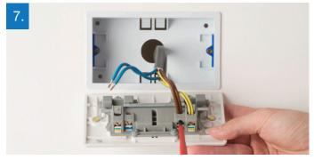
Whichever wiring configuration you find, unscrew each terminal screw to release the wires. You should now be able to remove the socket and place it to one side.
