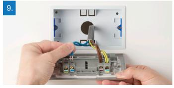
Place the blue wire(s) into the neutral terminal, brown wire(s) into the live terminal and the green/yellow wire(s) into the earth terminal. The terminals on the socket are colour-coded to help locate the correct one.
