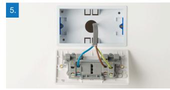
There will generally be three different wiring configurations. This photo shows a single wire of each colour connected to each terminal.
