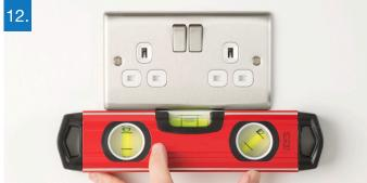
Insert and tighten the retaining screws provided. Use a spirit level to make sure that the socket is level. Restore the power at the consumer unit and test. For your safety, this product must be installed in accordance with local Building Regulations.
