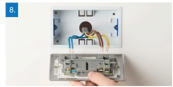
Line up the new socket and take note of where each terminal is located.
