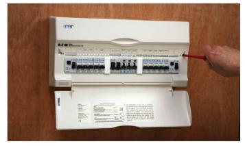
**Step 6 – External identification labels and fitting of main cover** The external circuit identification labels are now applied. The cover is then replaced easily and quickly using the quarter turn fasteners.
