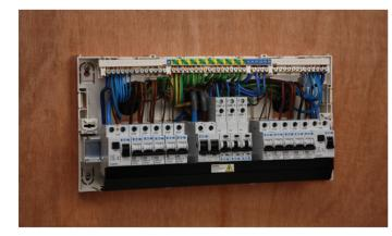
**Step 5 – Completion of internal wiring and labelling** Once all wiring is completed, the push-fit busbar cover is slotted into position and the internal labels can be applied.
