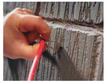
Slide the Linian Clip over the cable, so that it is seated in the rounded area.
