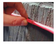
Compress the Linian Clips legs and simply insert into the hole by hand.
