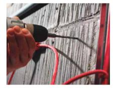
Drill 5.5mm diameter hole into the required material.
