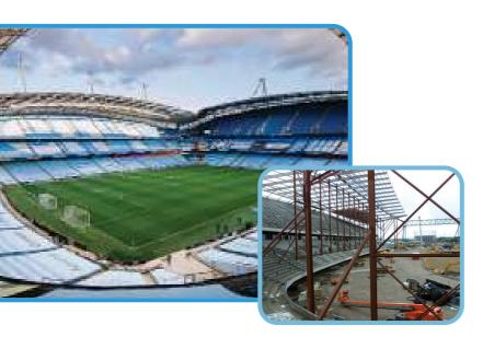
The stadium was designed and engineered by Arup and built by Laing Construction at a cost of £112m. The design includes a cable-stayed roof structure entirely supported by 12 exterior masts and cables. The stadium design has received many accolades, including a 2003 special award from the Institution of Structural Engineers for its unique structural design and a 2004 award from the Royal Institute of British Architects for its innovative building design.
