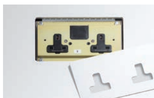
ADD FRONT PLATE ADJUST AND FINISH
