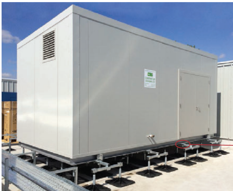
Typical plantroom support utilising 8no. F-QUAD-500-A
