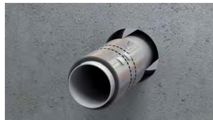
3. Bend and lock the tabs
