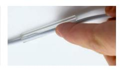
6 Attach cable clips underneath cabinet to discreetly secure the cable in place.
