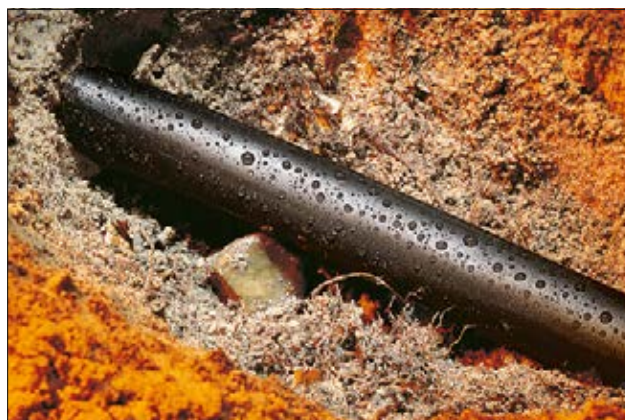
TREDUX HA47 - application below ground.
