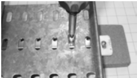
3) An electric screwdriver is used to fix the tray to the bracket the Thread Forming Screw.
