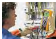
Insulation test at a distribution panel
