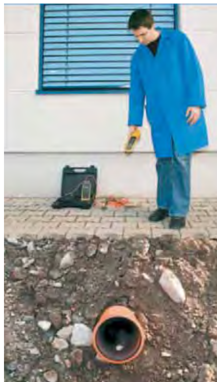
Locating cables and pipes in the ground
