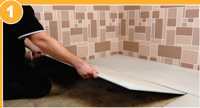
1 Fit the ECOMAX Insulated Tile Backer Board to the floor securely following the manufacturers instructions.
