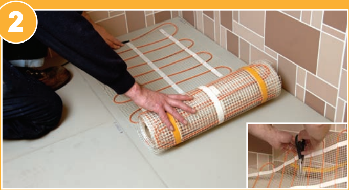
2 Roll the mat onto the floor. When you reach the end of a row, cut the backing mesh and turn the mat through 180° and position the next strip adjacent to the first.
