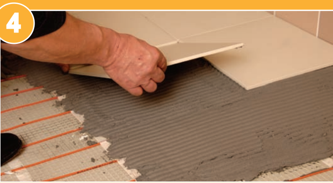
4 Cover with a layer of self-leveling compound/flexible tile adhesive and allow to dry before tiling. Alternatively lay the adhesive and tiles in one step ensuring the cable is totally encapsulated to prevent air gaps.
