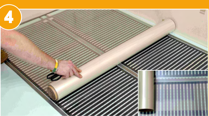
Cover the total ECOFILM SET installation with POLYESTER VAPOUR BARRIER (available separately).
