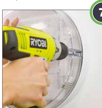
Use captive screws to screw the diffuser into place
