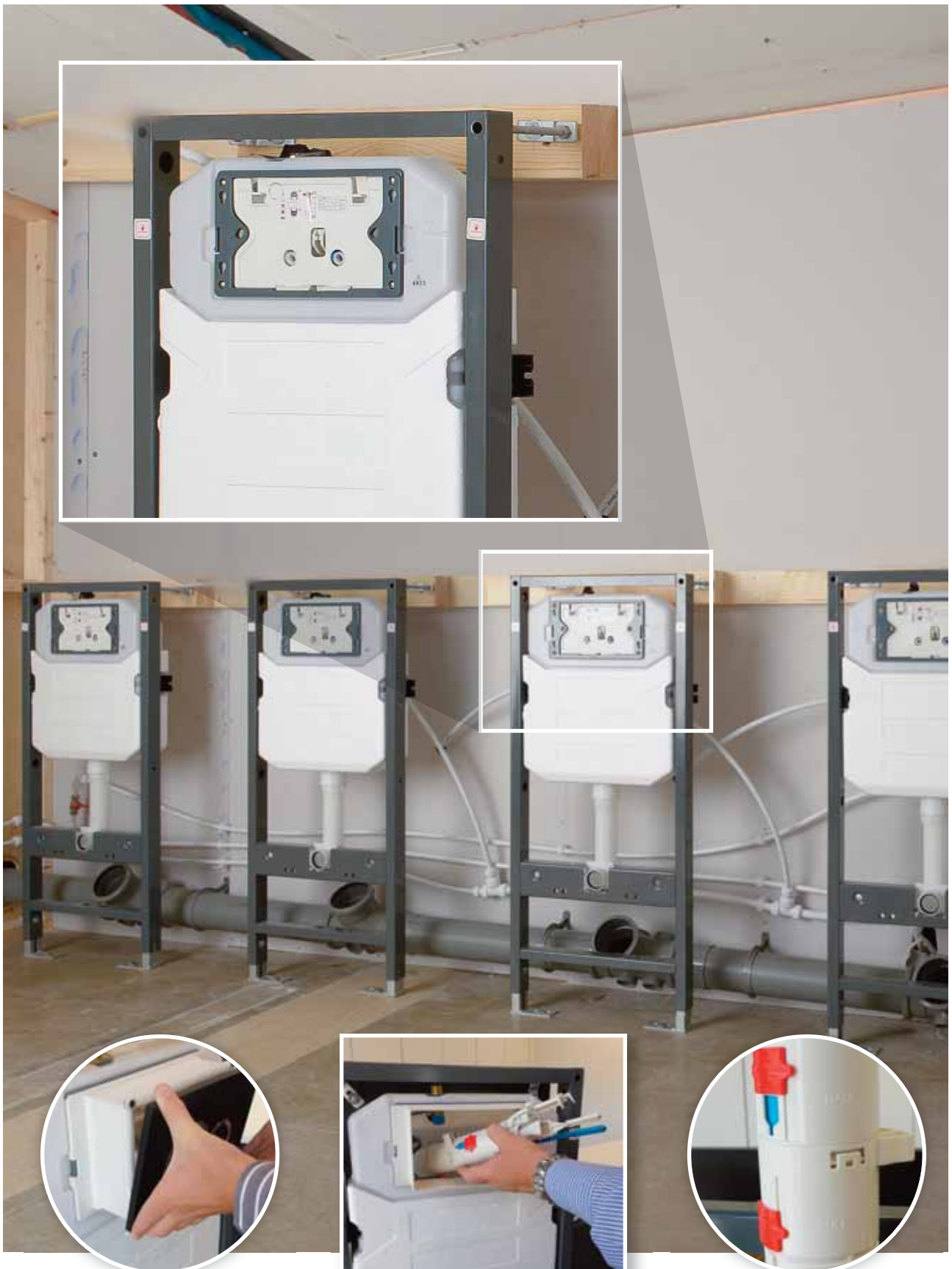
Front plate removed from the front of the unit
