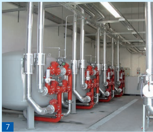
7 Water filtration / softening system for commercial applications
