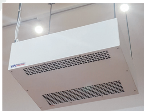
SMH heater suspended from drop rods
