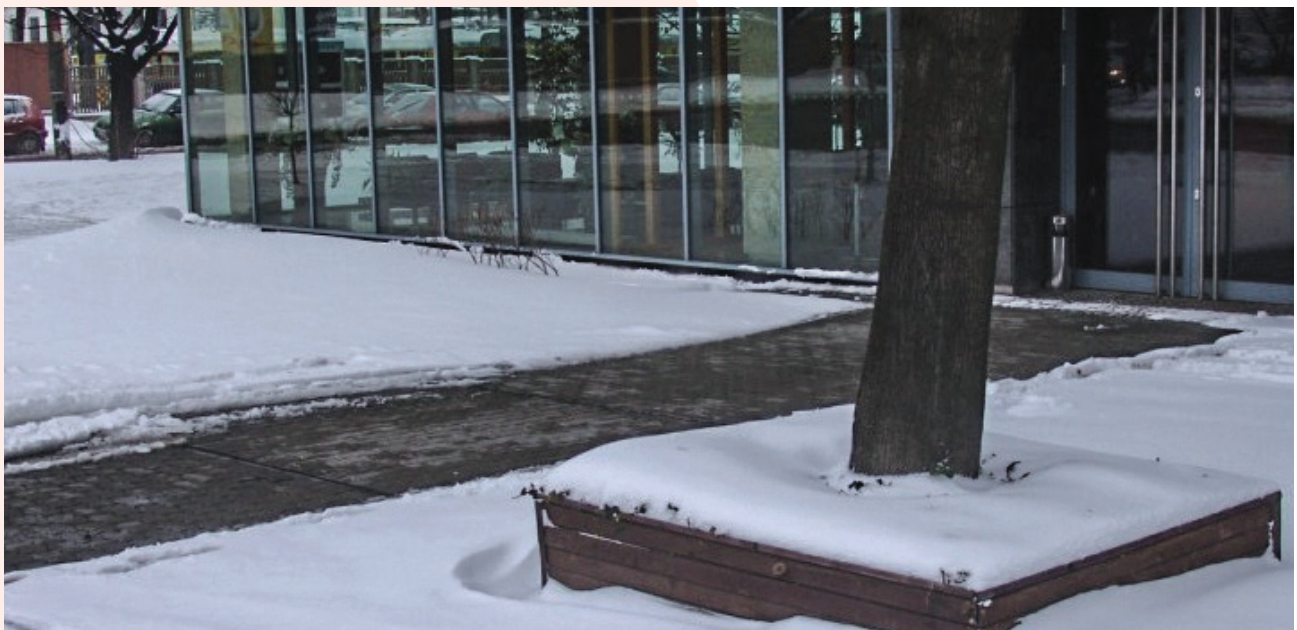
ERC Snow and Ice Melting Mat providing safe access to an office building
