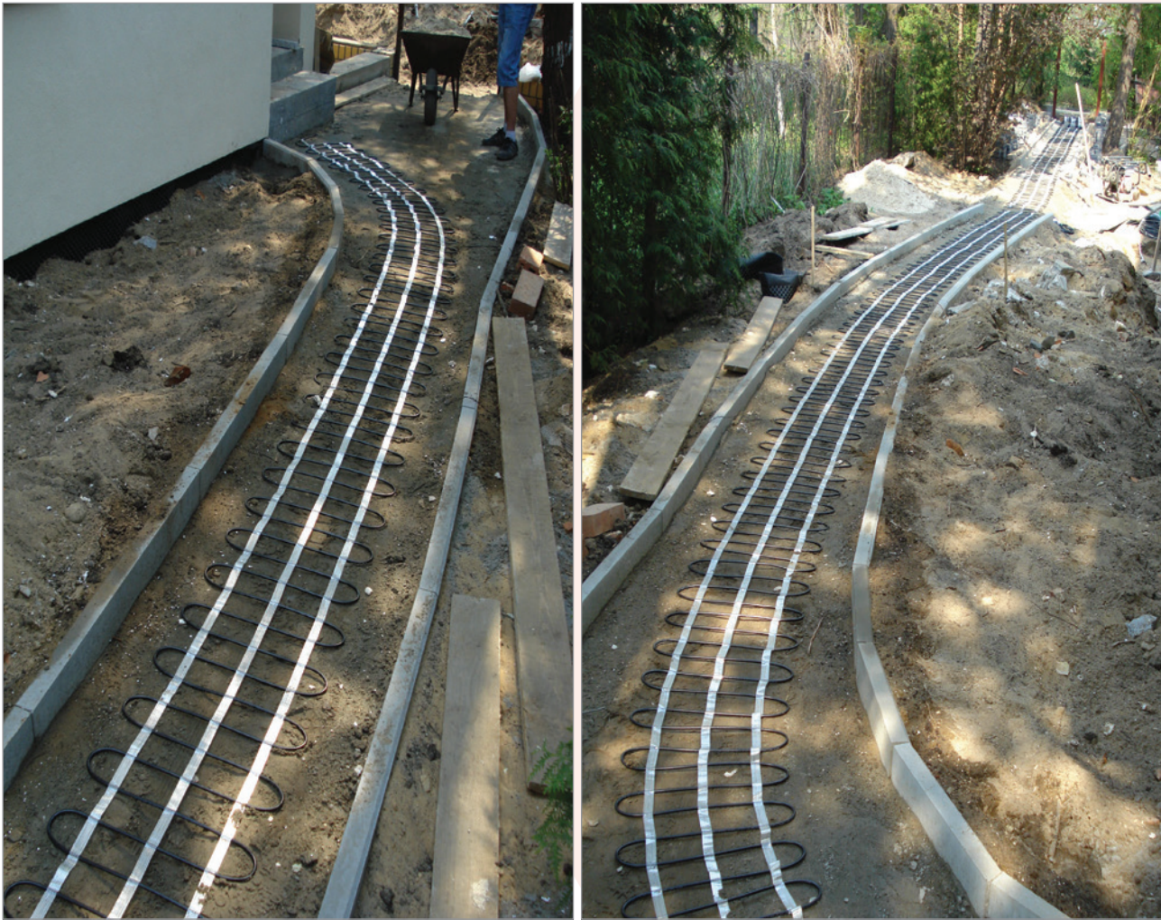
ERC Snow and Ice Melting Mat prepared for concrete pour
