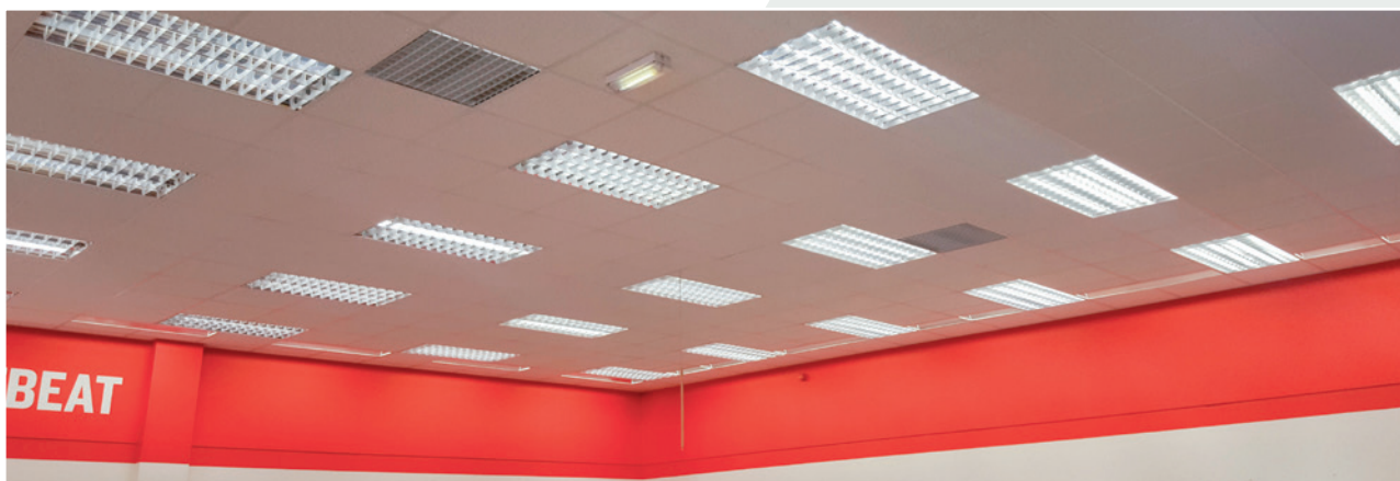
Multiple heaters installed in a large showroom
