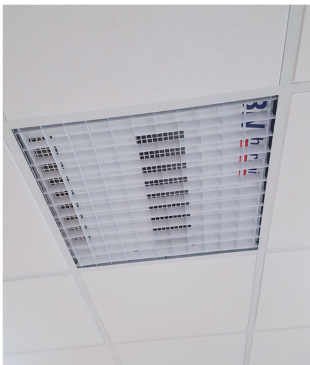
Heater specifically designed for integration into a suspended ceiling grid
