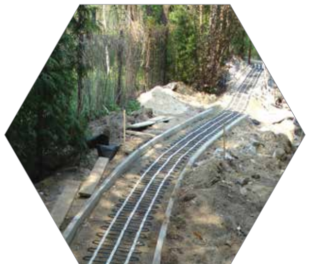
ERC Snow and Ice Melting Mat prepared for concrete pour
