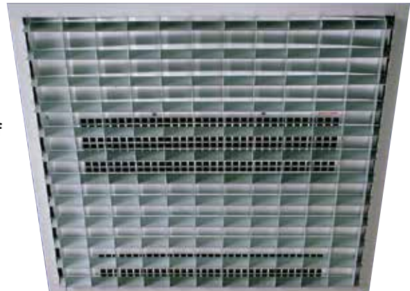
CHS heater installed in a 600 x 600 ceiling grid as part of a multi-heater system
