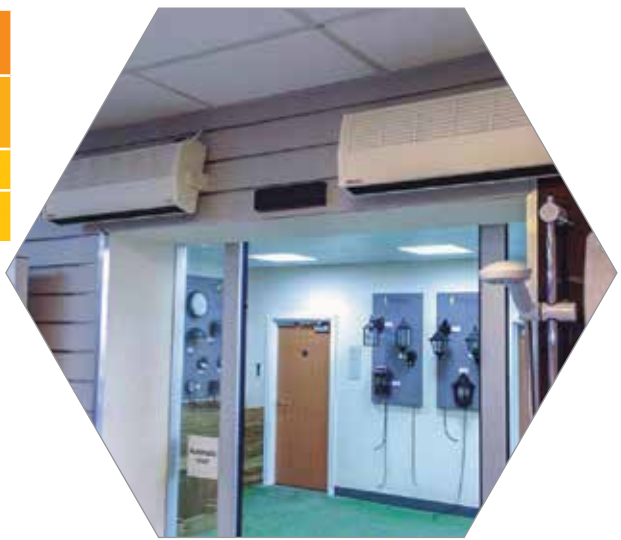
830T installed over a showroom door
