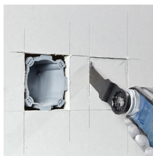
Problem-free plunge cuts in plasterboard
