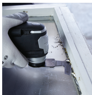
Cutting window putty (sealing compound)
