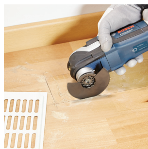
Cutting out laminate/parquet accurately, e.g. for installing a ventilation grille
