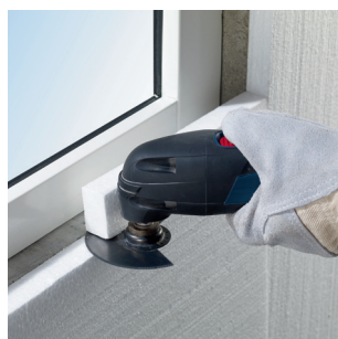
Flush cutting protruding insulation material, e.g. polystyrene
