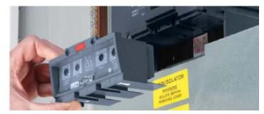
Important Note: The incoming switch unit is supplied fitted in all the Powerstar 250 range. The user only has to select and fit the appropriate trip module (with or without protection)
