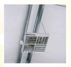
Two destratification units were installed to enhance economy. These devices are suspended from the roof and recirculate warm air that would otherwise accumulate at high level. It is estimated that the use of destratification units reduces heating bills by approximately 30%.
