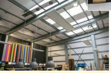
Whilst the radiant cassettes provided the main source of heat, they were augmented by a commercial air curtain which created an invisible barrier across the entrance preventing valuable warm air from escaping.
