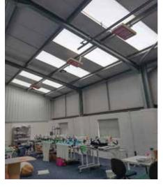
When using an industrial sewing machine, it is vital that the operator can accurately match colours of fabrics and threads. For this reason, halogen heaters from BN Thermic's Magic Lamp range were selected. These heaters provide all the performance associated with a conventional halogen heater but without the familiar red glow.
