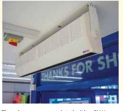
The scheme was completed with a 6kW overdoor heater to provide a warm welcome for customers
