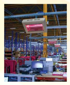
This distribution centre is far too large to consider installing a conventional heating system. However, there was a requirement to provide instant, direct heat to 53 individual packing stations. BN Thermic surveyed the site and recommended 1.5kW halogen heaters using the latest Magic Lamp technology. These heaters provide all the performance associated with conventional halogen heaters but with the light output reduced to a barely discernible glimmer.
