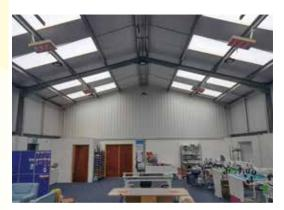
The halogen heaters were suspended at high level and arranged in an evenly distributed grid.
