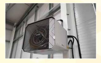
This was a classic industrial project where fan heaters and destratification units work together to heat a building and keep running costs to a minimum.
