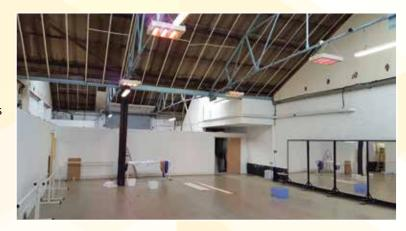
The solution was to suspend a grid of four halogen heater from the ceiling. The positioning of the heaters was carefully considered to ensure an even distribution of the radiant effect and control was provided by BN Thermic's MC1 control panel which provides an easy means of adjusting heat intensity.
